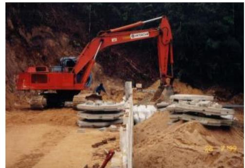
**Fig. 13 : Laying of the galvanised reinforcement tendons.**
