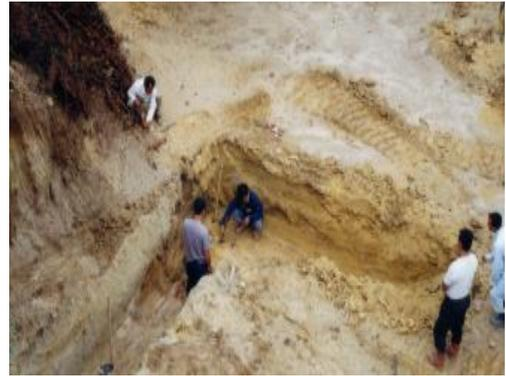
**Fig. 11: Gravel wrapped with geotextile is placed into the excavated trench to form Rock Fill.**
