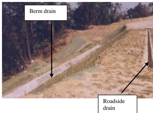
**Fig. 16 : Completed RE wall with berm drain and cascading drain.**
