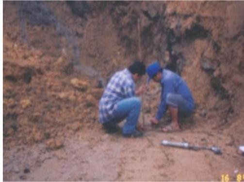
**Fig. 10 : Trench is excavated at the toe of RE Wall to construct the Rock Fill.**
