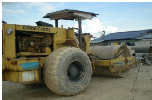
Figure 1: Measurement of background noise level when equipment (compactor) was off
