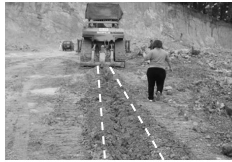
Figure 2: Cut groove produced by ripper dozer
