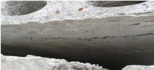
Figure 7: Crack in HCS
