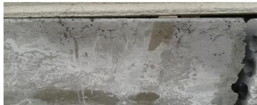
Figure 5: Pore defect
