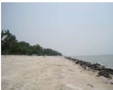
Figure 1: Pantai Remis in Kuala Selangor district is facing erosion problem that requires coastal defence work to curb it.
