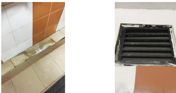
**Figure 3** Unclean ducting system and stained floor, ablution room Gate-B
