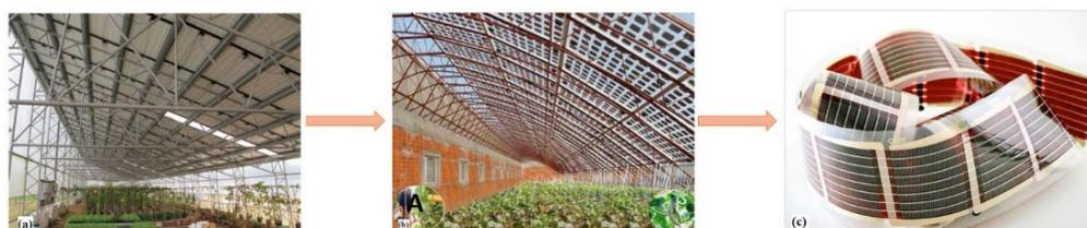
**Figure 1.** Revolution of PV technology (a) crystalline silicon modules (Castellano et al., 2016), (b) thin film amorphous modules (Hassanien et al., 2016) and (c) OPV (ApS, 2020)
